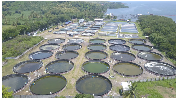
Fig. 7. Circular ponds in Situbondo, north of Banyuwangi, which enable more effective sludge collection. Picture: © MMAF, from Bulkini (2021)
